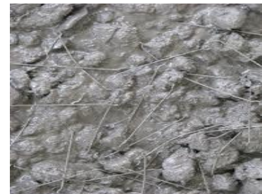
Figure 2: Steel fibers in fresh concrete
